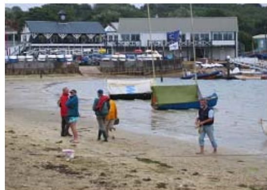
Setting-out for Baywatch restaurant. Picture by Steve Bradwell
